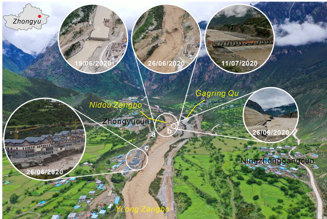
Figure 12. Examples of GLOF damage to downstream infrastructure and buildings at the confluence of Nidou Zangbo and Gagring Qu. Background aerial photo by Heng Li taken on 26 June 2020. (a) Comparison of the bridge connecting Zhongyucun and Ningzhonggangcun before, during (photos: Heng Li), and after the GLOF (rebuilt, photo: Kejun Ma). (b) Destroyed roads (photo: Heng Li). (c) Affected buildings at risk (photo: Heng Li).
