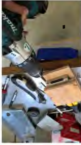
(b) Drilling larger screw hole.
