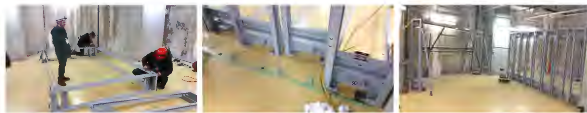
Figure 5-7: Assembly of B2 chassis.
