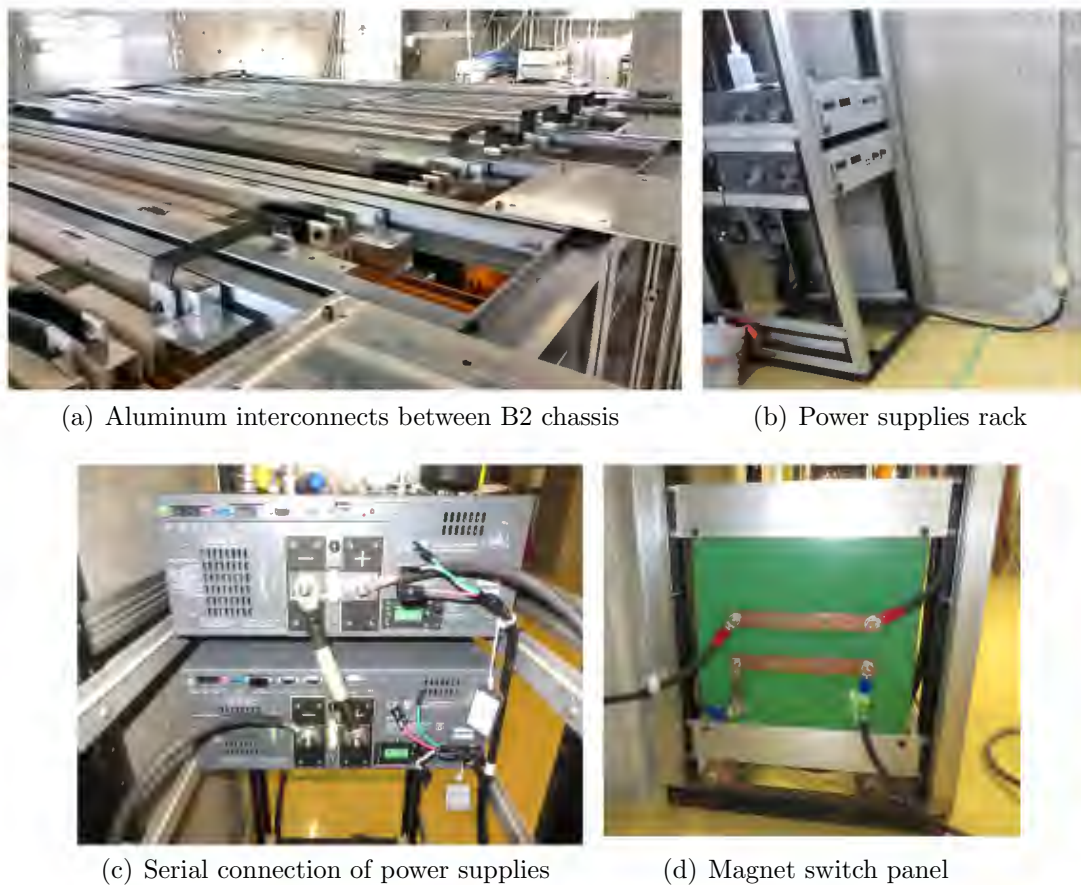
Figure 5-15: Magnet connection details.
