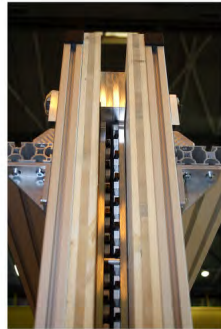
(f) Bolting the four corners.
