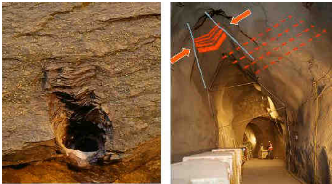
Figure A.4-21. Buckling of strata in a borehole (left) and geologically-induced overbreak in a gallery of the Mont Terri URL (right; with mechanism indicated; hatched = bedding planes).
