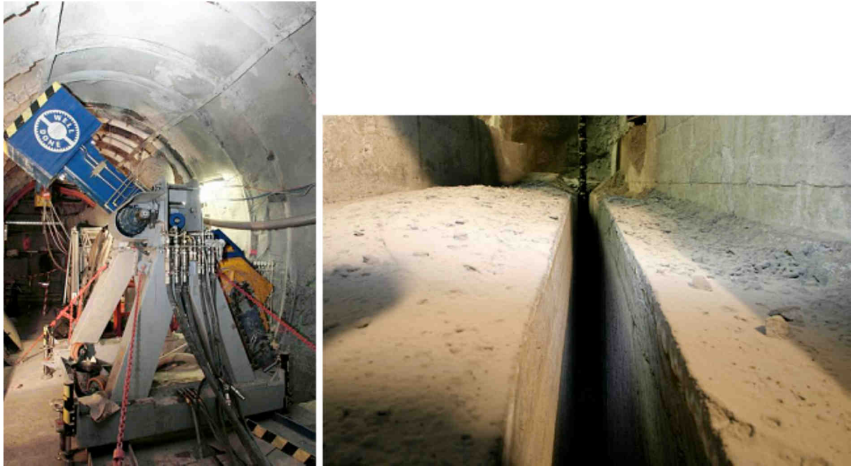
Figure 3-52. Saw cutting of a 7 cm wide slot in the Bure URL (out of Andra 2005b)
