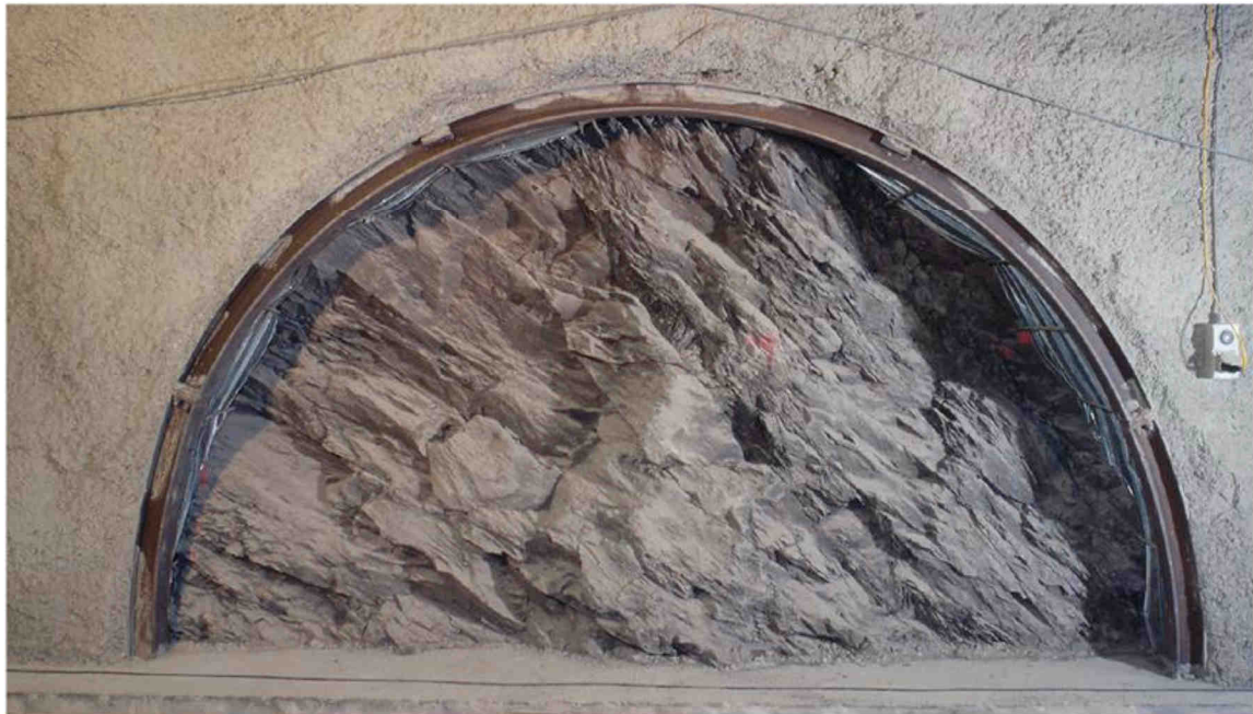
Figure 2-4. Illustration of the Main Fault in Gallery 98 at Mont Terri Top: Photo view, © Comet, Zurich - Bottom: Structural geological interpretation (from Nussbaum and Bossart 2008)
