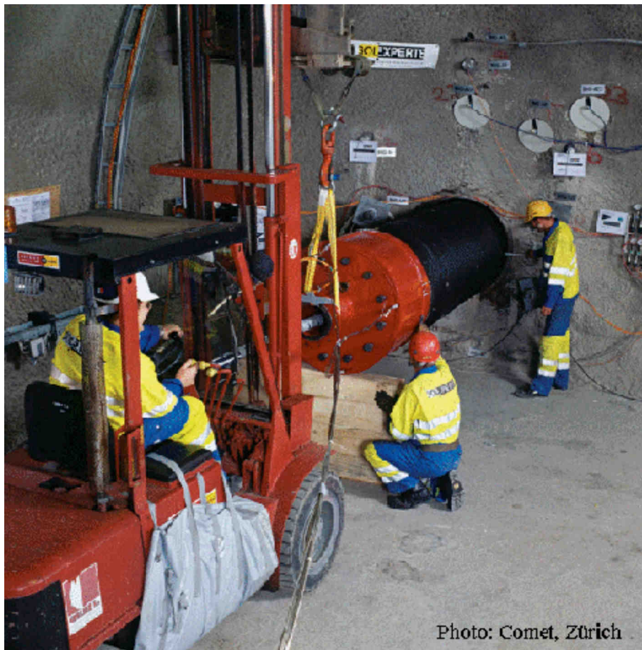
Figure 3-36. HG-A Experiment: Emplacement of the megapacker (from Marschall et al. 2008c)
