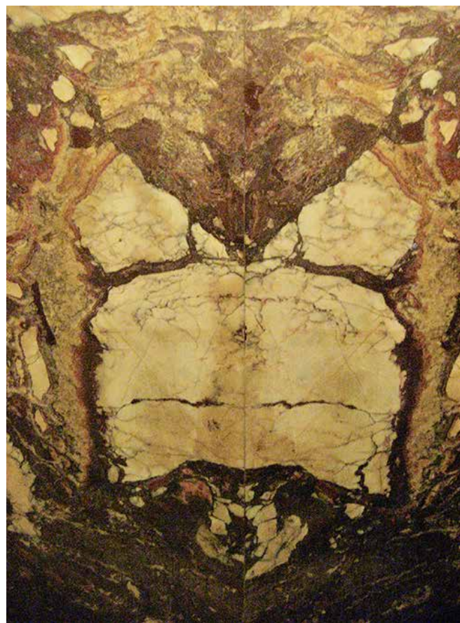
10 Adolf Loos, Goldman & Salatsch Building (Looshaus), detail of marble wall cladding at the Herrengasse entrance, 1909–1911, Vienna
