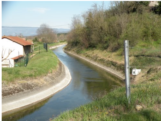
Figure 2.11 – The La Bourne irrigation canal ( Valence in France).
