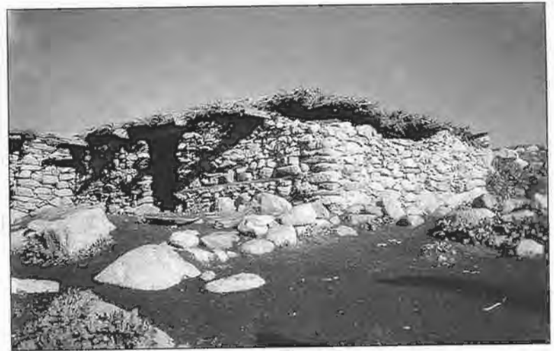
Transitional houses of transhumant herders (Ajars) without proper doors or plastering
