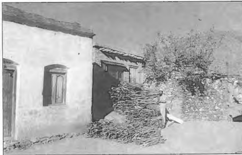
Wood and stone are being replaced with brick and cement as construction material.
