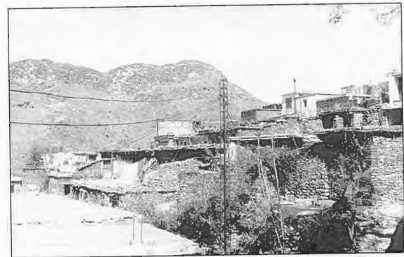
Traditional housing pattern can still be seen on the hillside slopes in narrow side valleys.
