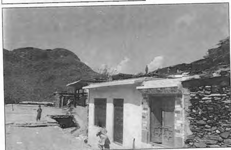
From tradition to modernity: stones are being replaced with bricks in house construction
