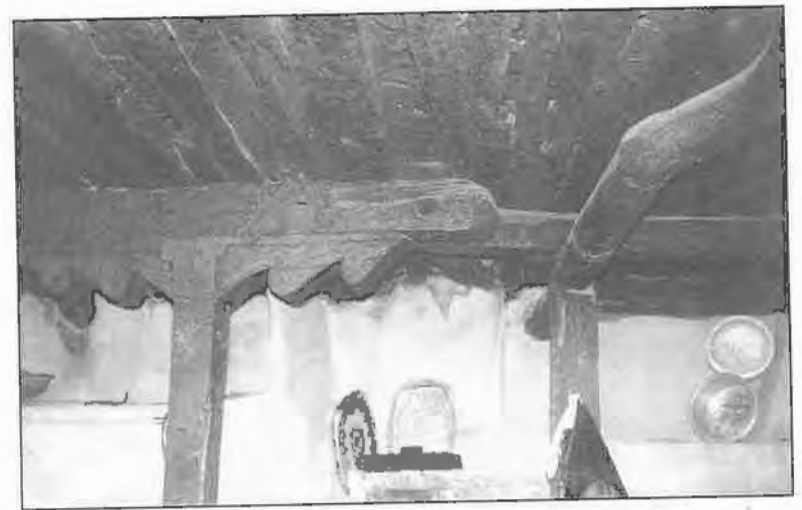
Wooden beams and carved pillars inside a traditional house
