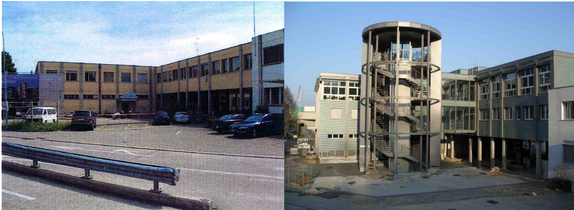
Figure 1: Studied building before and after renovation (source: P. Previdoli)
