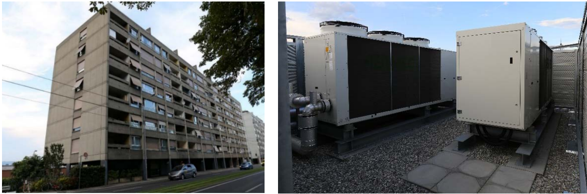
Figure 1. Studied collective multifamily building (left) and industrial air-source heat pumps (right)
