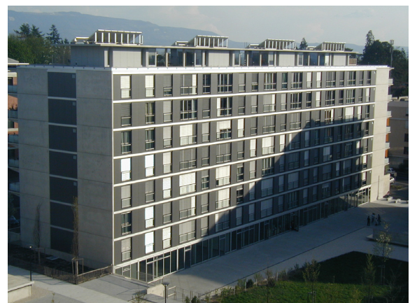
Figure 3: Solar collectors and accessible roof on Gardiol building (NW).
