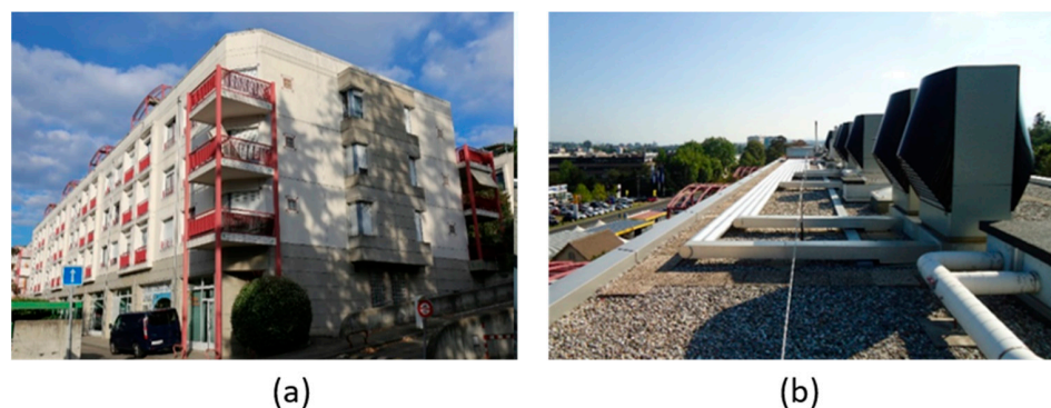
Figure 4. Hybrid ASHP system. (a) Non-retrofitted MFB and (b) six air-to-water heat pumps on the roof.
