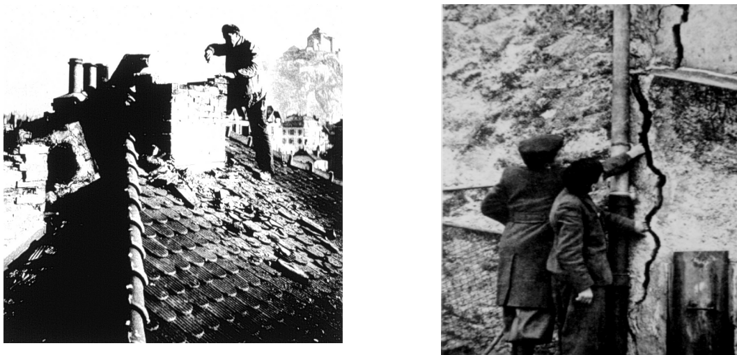
Figure 1.9. Damages on buildings. Left side, a chimney was partially destroyed (Sion area; Mr J.-D. Rouiller's collection). Right side, fissure on a wall (revue L'illustré, 1946).
