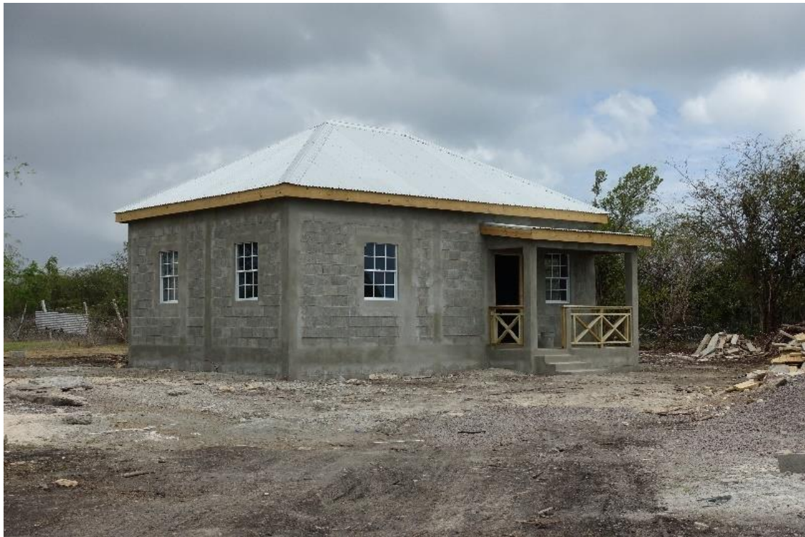
As the grey clouds roll across Barbuda, signalling the beginning of the 2021 Atlantic hurricane season, UNDP-led construction crews have finished another house under the EU-funded housing scheme. The squarely built homes lacking finishing touches stand in stark contrast to their larger neighbours. Delays and decreases in the program have led to political polarization as desperate families without durable solutions seek entry into the already decided pool of recipients. Codrington village, Barbuda (Marazita, May-2021).
