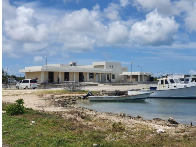
The fisheries building stands, with its concrete façade and flat roof, in stark contrast to neighbouring structures. The building was one of few structures to survive Hurricane Irma and served as a community centre in the days following landfall as Barbudans awaited evacuation. Codrington village, Barbuda, Antigua & Barbuda (Marazita, Jun-2021).
